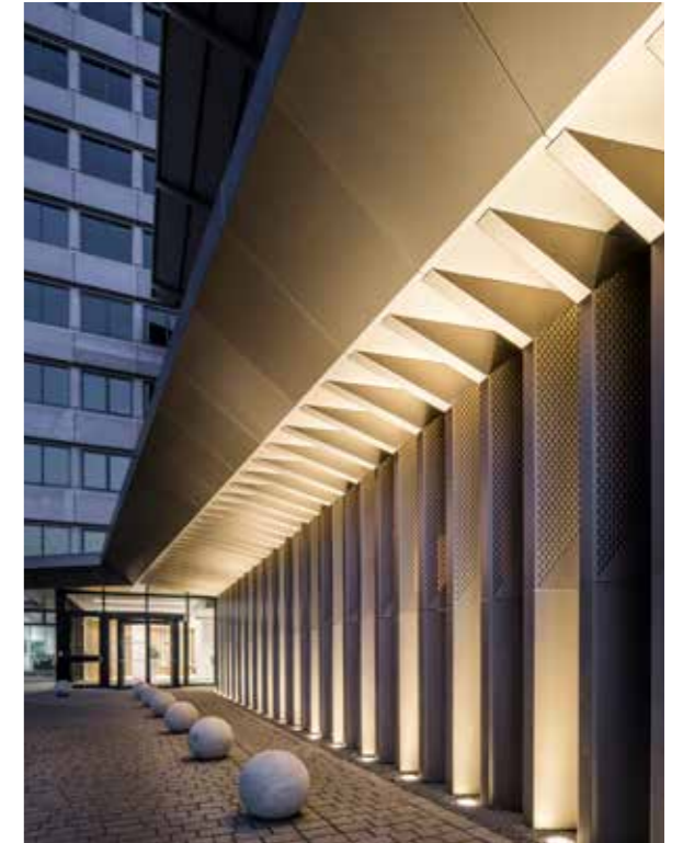
The Switch entrance.
