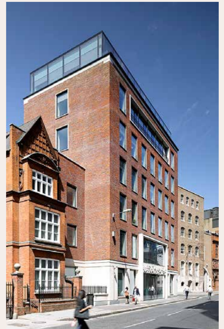
St Paul's House entrance on Warwick Lane.
