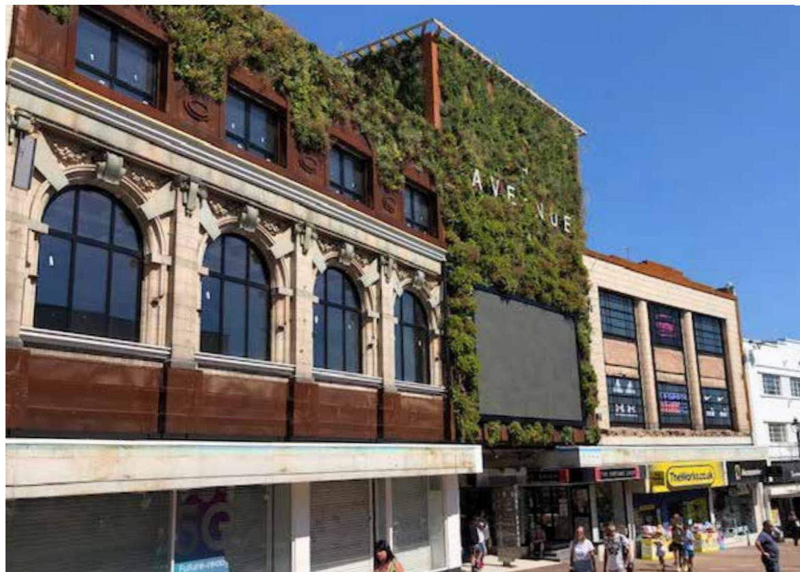
Commercial Road facade.
