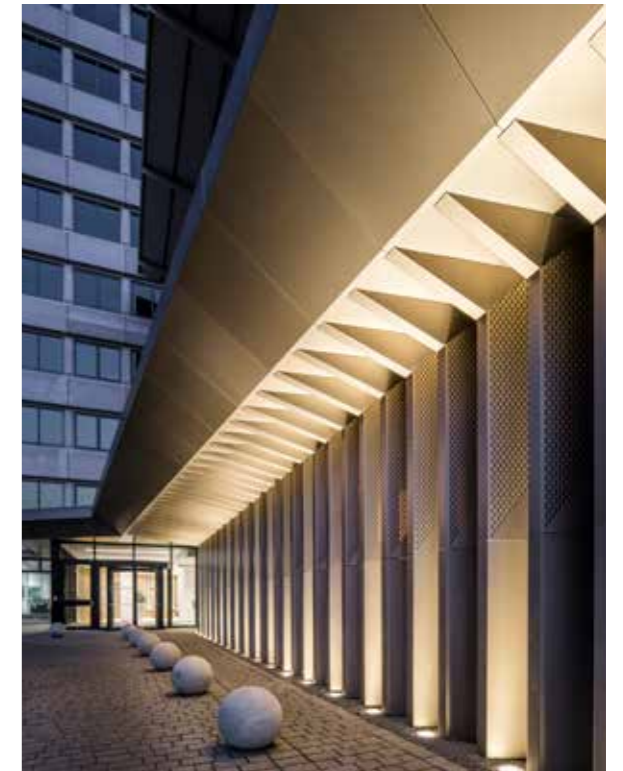
The Switch entrance.
