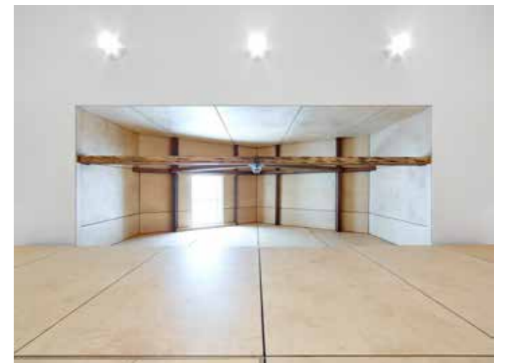
The creation of a new light well opens up a portion of the roof space, providing a brighter, more voluminous feel.
