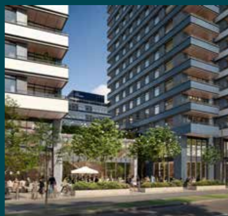
Tolworth Tower London
