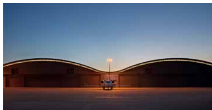
Industry & Technology / Farnborough Airport Hangars.
