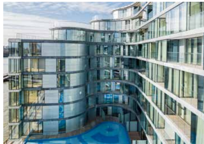
The whole building is clad in unitised curtain walling and provides 61 residential units, 97 serviced apartments and 930m 2 of retail.
