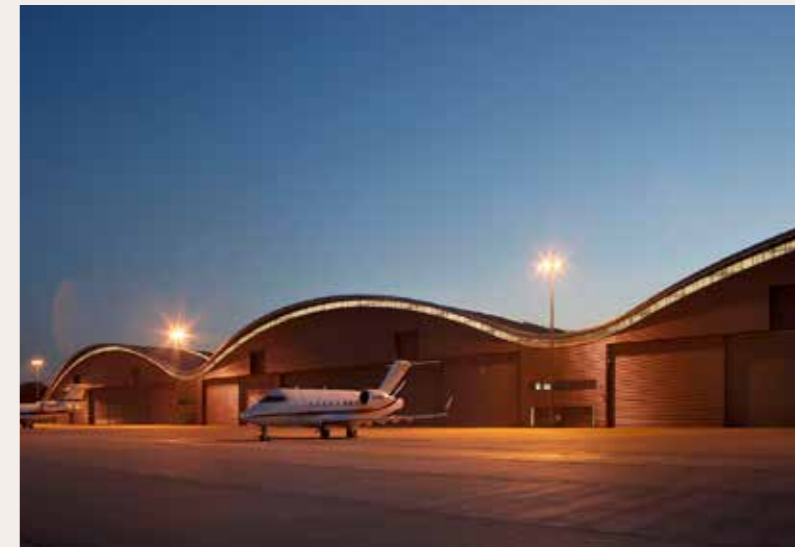
Farnborough Airport Hangars.
