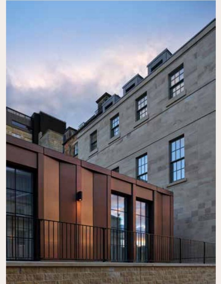
Townhouse extension and copper clad pavilion.
