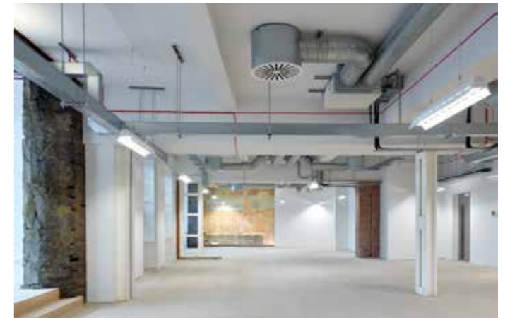
A key driver underpinning the scheme is to expose and enhance the historic fabric of the existing building to create character speculative office floorplates.
