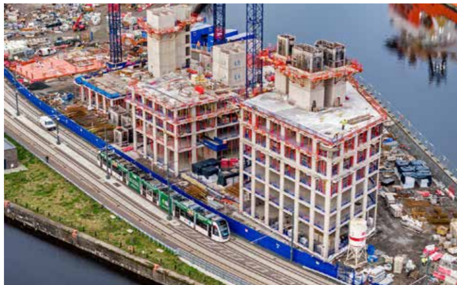
Currently under construction (2024).
