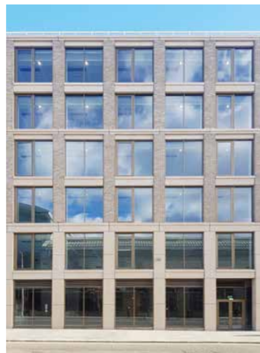
No2 Freer Street office facade.
