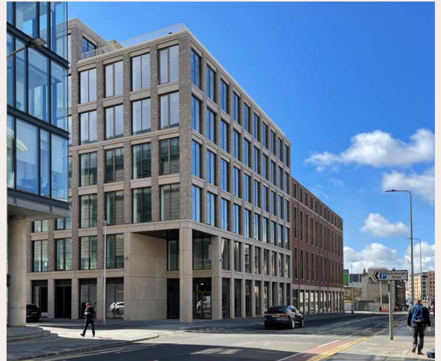
No2 Freer Street flexible Cat A office space.
