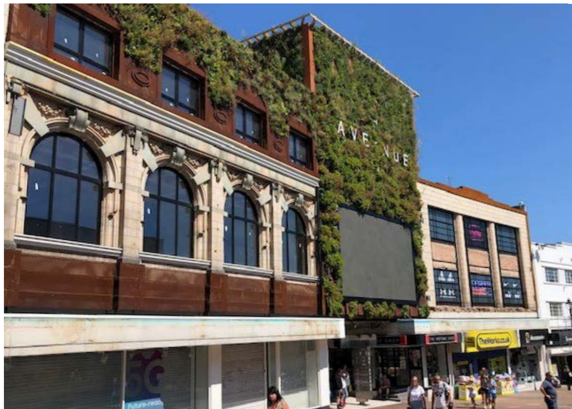
Commercial Road facade.
