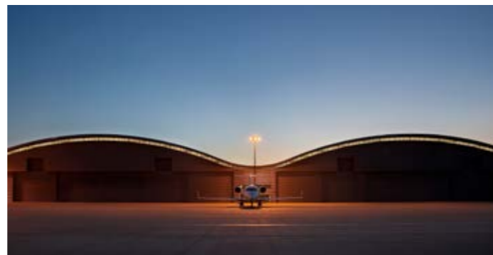
Industry & Technology / Farnborough Airport Hangars.
