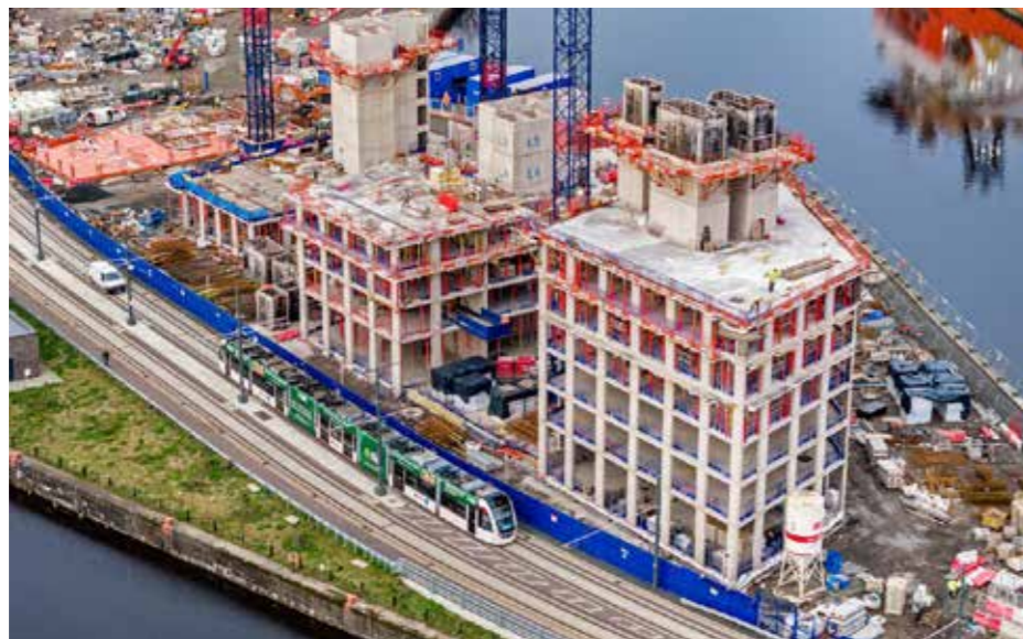
Currently under construction (2024).
