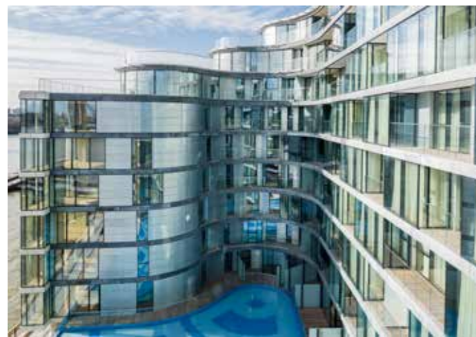
The whole building is clad in unitised curtain walling and provides 61 residential units, 97 serviced apartments and 930m 2 of retail.
