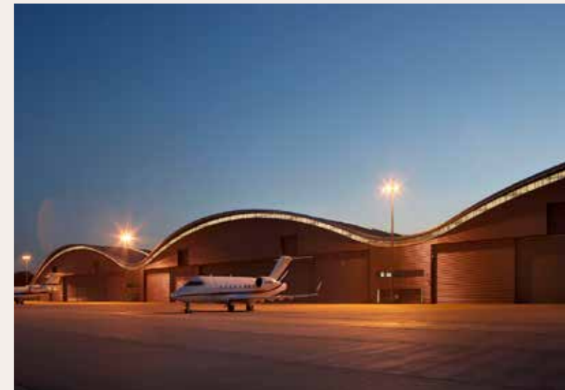
Farnborough Airport Hangars.
