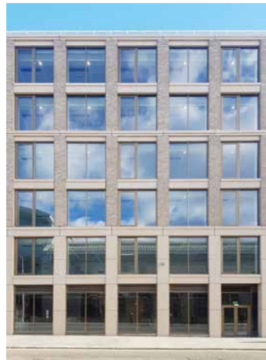
No2 Freer Street office facade.
