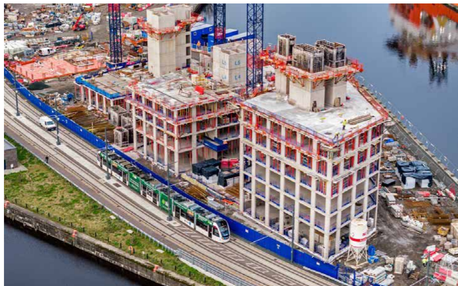
Currently under construction (2024).
