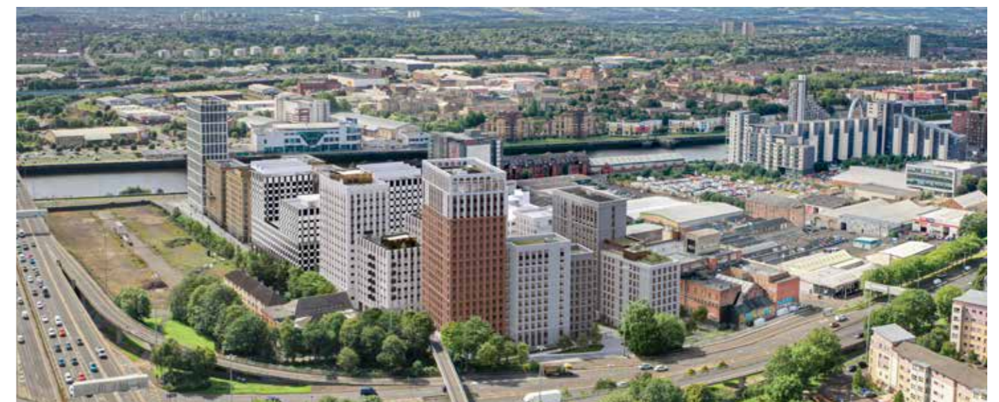
Aerial visual looking south.
