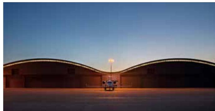
Industry &amp; Technology / Farnborough Airport Hangars.
