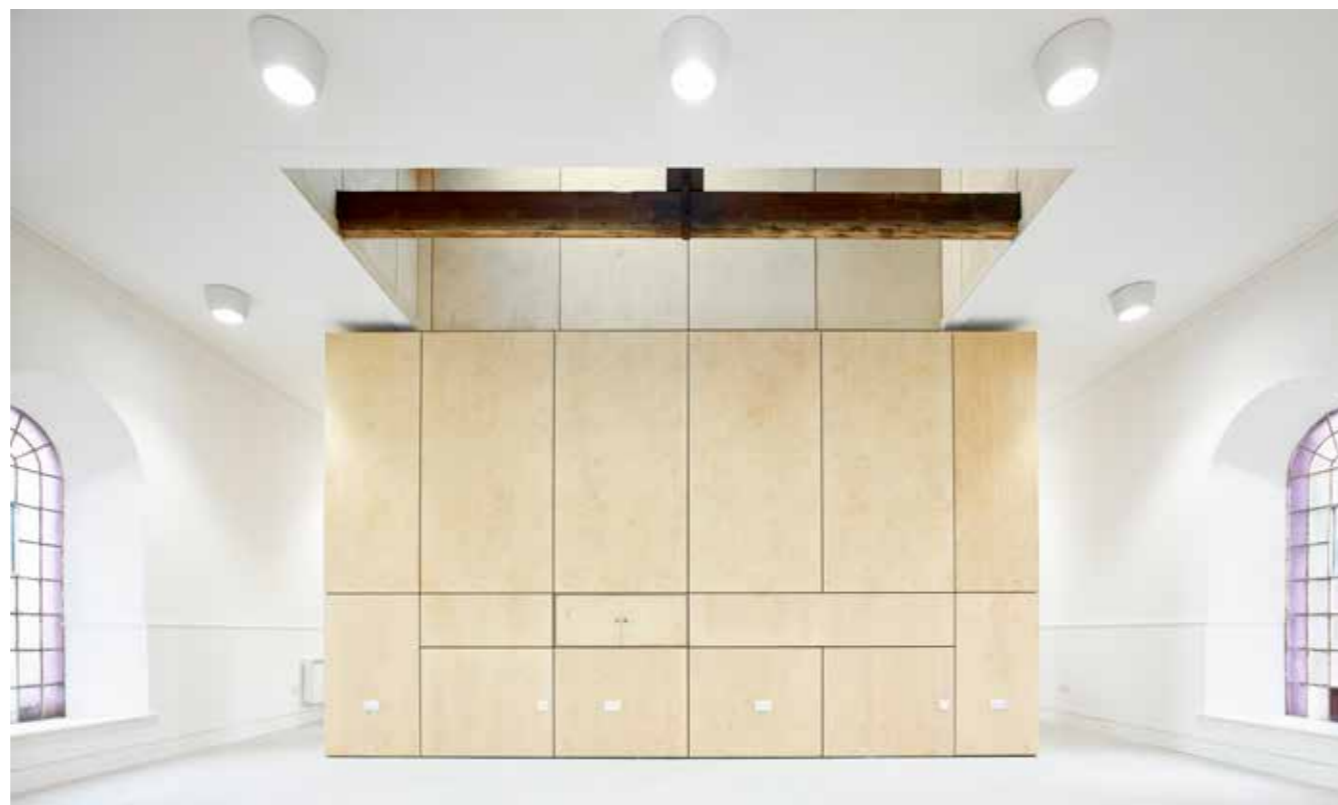
Re-imagined as a flexible community-use space: The levelling of the previously raked floor has facilitated a more flexible space, into which a birch plywood-lined volume has been inserted, containing key ancillary accommodation.
