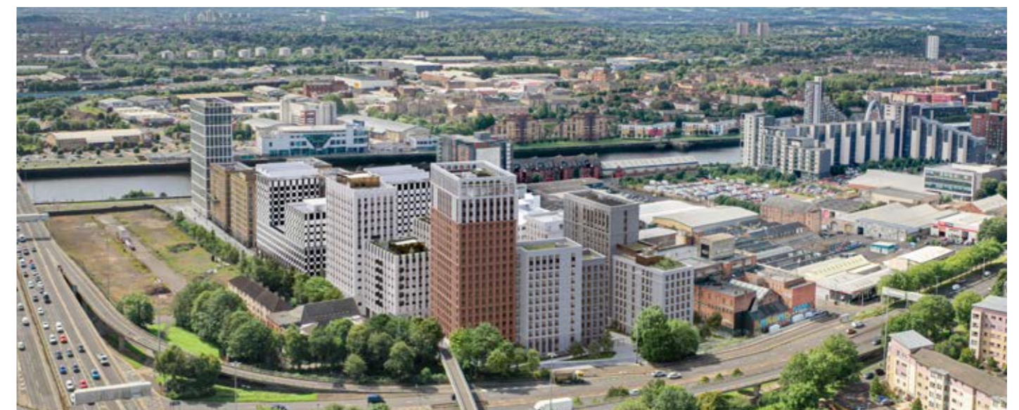
Aerial visual looking south.
