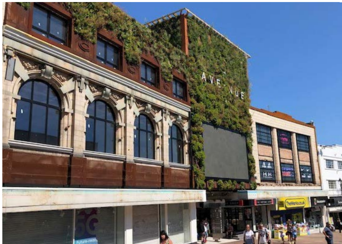
Commercial Road facade.
