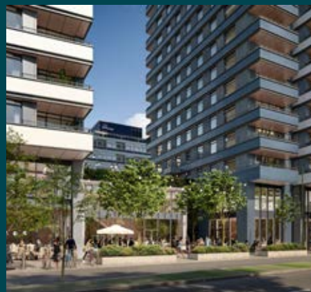
Tolworth Tower London
