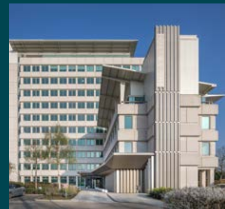
The Switch Slough
