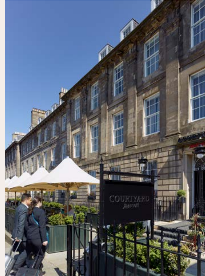
Scottish Property Awards 2018, Development of the Year Commercial Buildings (Highly Commended).
