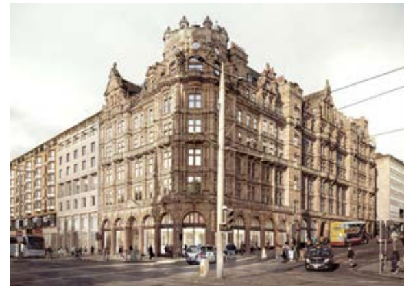
Corner view of the building looking towards the Princes Street entrance and South St David Street entrance.
