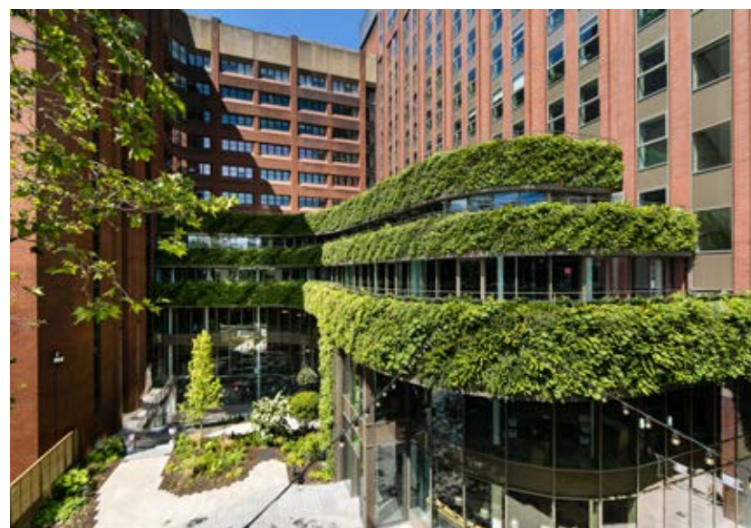
View from the courtyard.
