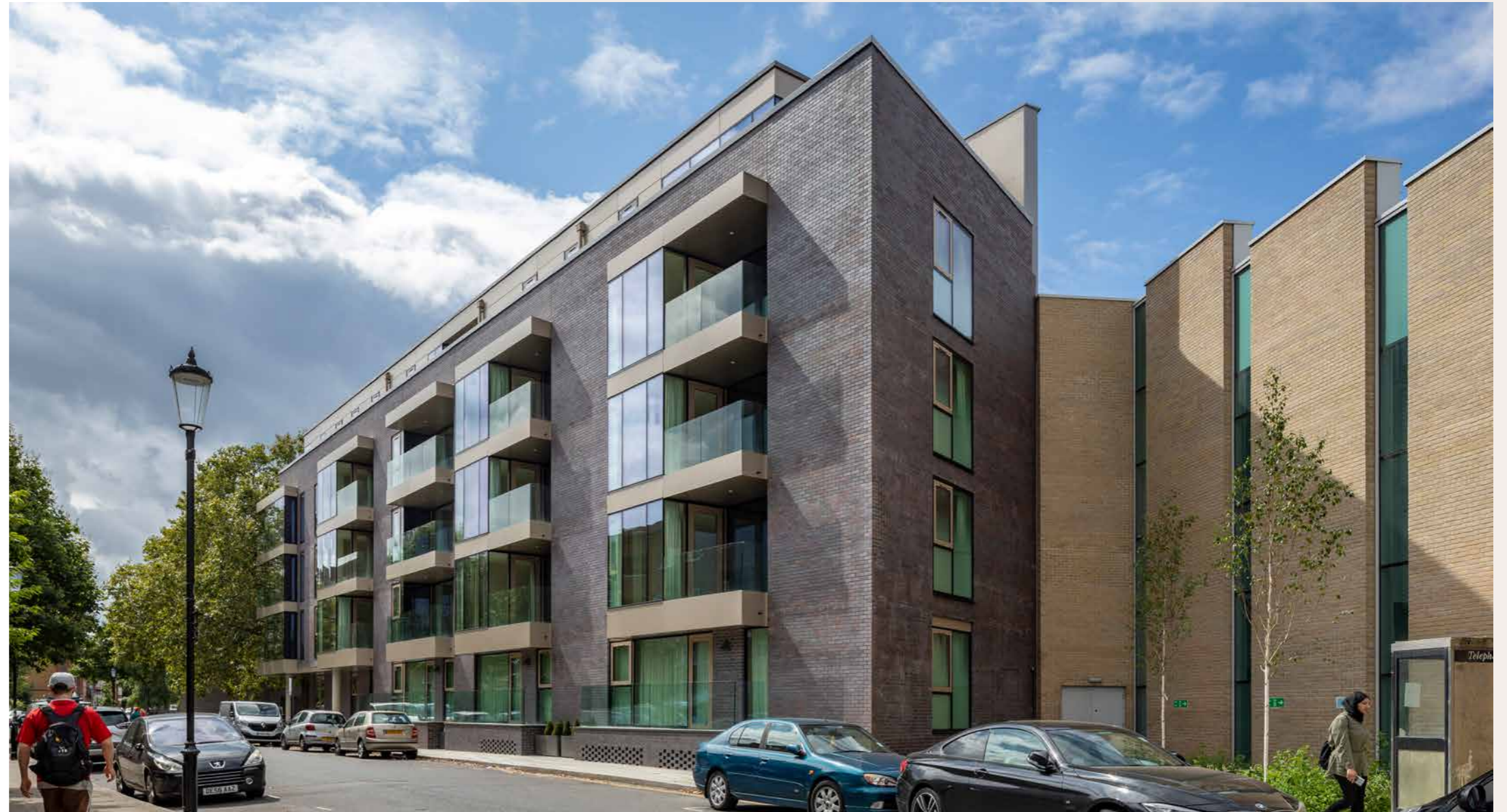
Kensington Academy apartments.
