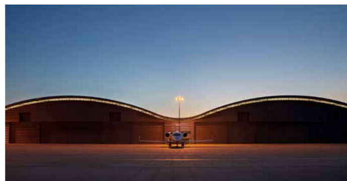
Industry & Technology / Farnborough Airport Hangars.
