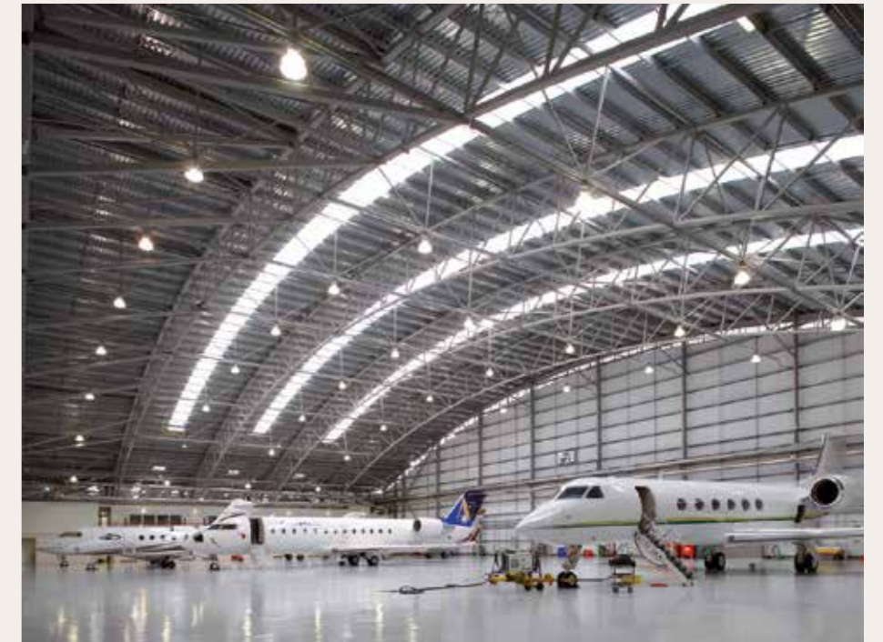
The maintenance and hangar facilities are column free, utilising an innovative design created in tandem with the structural engineers, Buro Happold.
