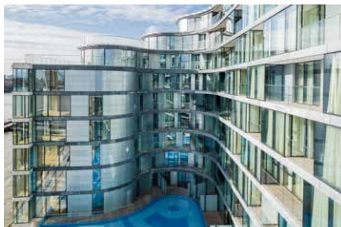
The whole building is clad in unitised curtain walling and provides 61 residential units, 97 serviced apartments and 930m 2 of retail.
