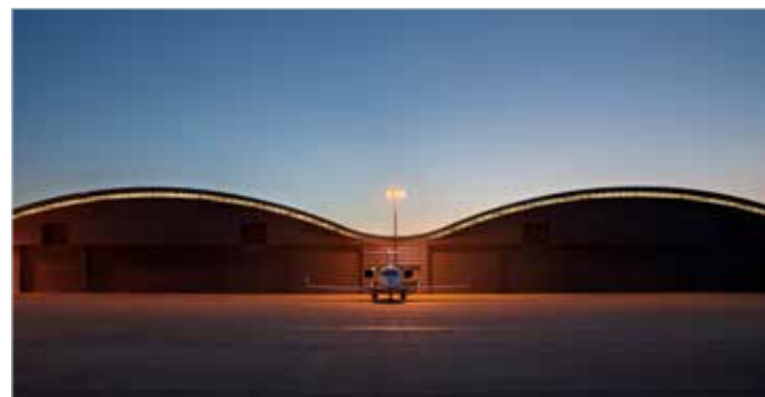
Industrial / Farnborough Airport Hangars.
