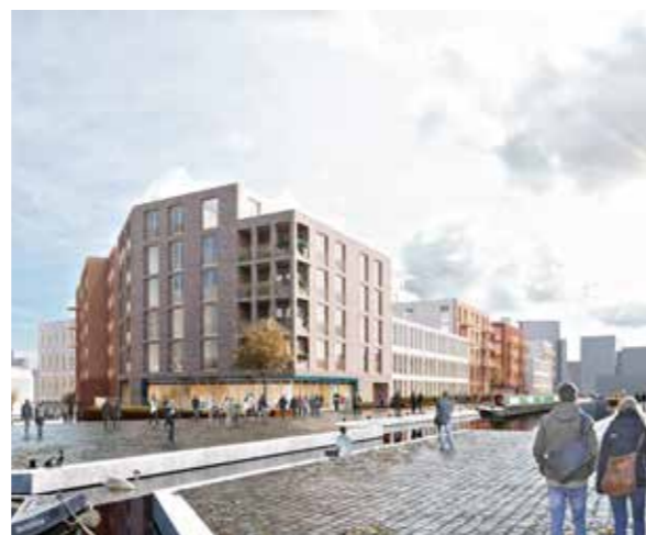
View from Leamington Lift Bridge.
