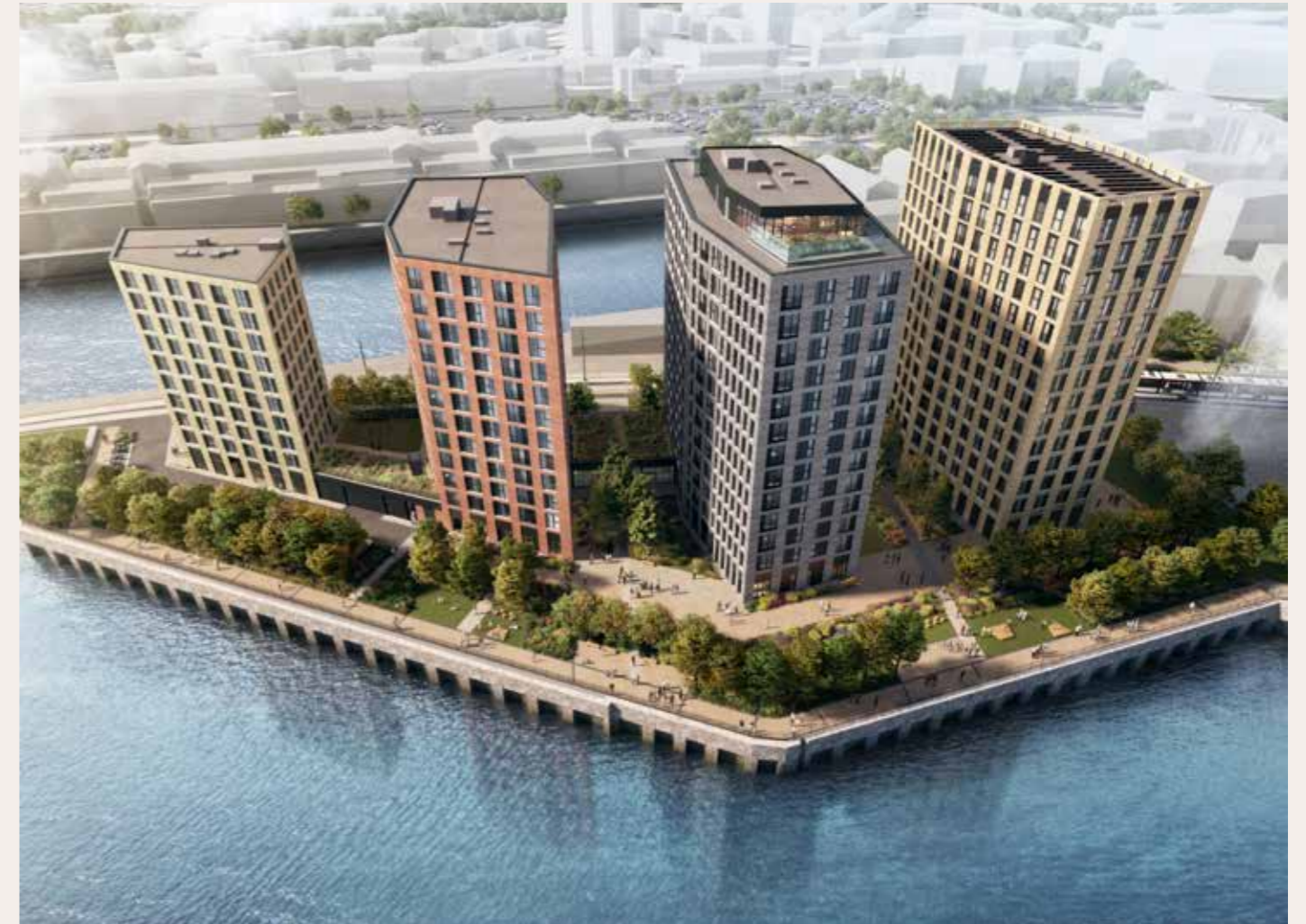
Aerial view of Dockside.
