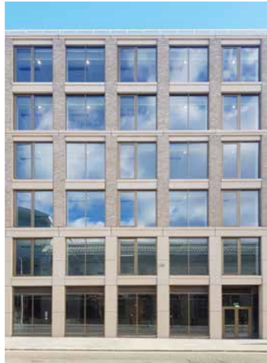
No2 Freer Street office facade.
