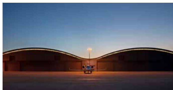
Industrial / Farnborough Airport Hangars.
