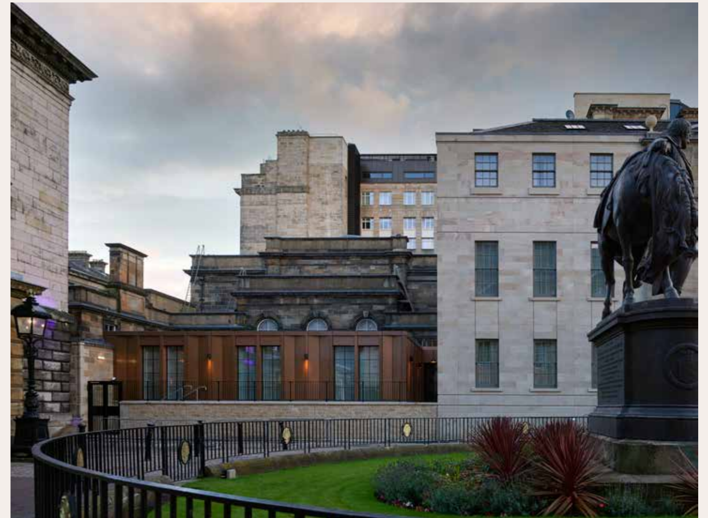
The Gleneagles Townhouse project both renews an existing building and extends it with a copper-clad 'pavilion' structure and a new masonry façade complementary to the setting.
