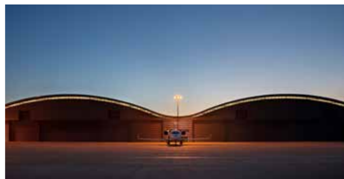
Industrial / Farnborough Airport Hangars.
