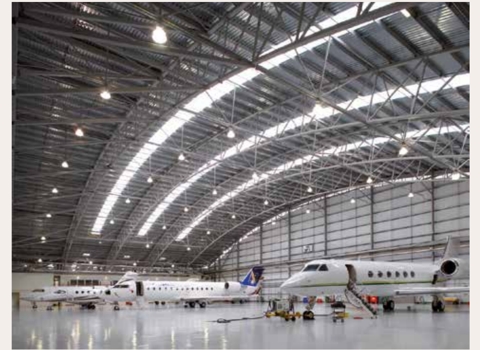
The maintenance and hangar facilities are column free, utilising an innovative design created in tandem with the structural engineers, Buro Happold.
