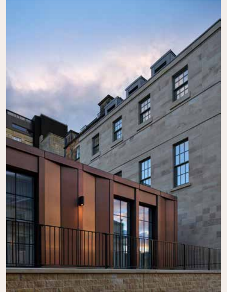
Townhouse extension and copper clad pavilion.
