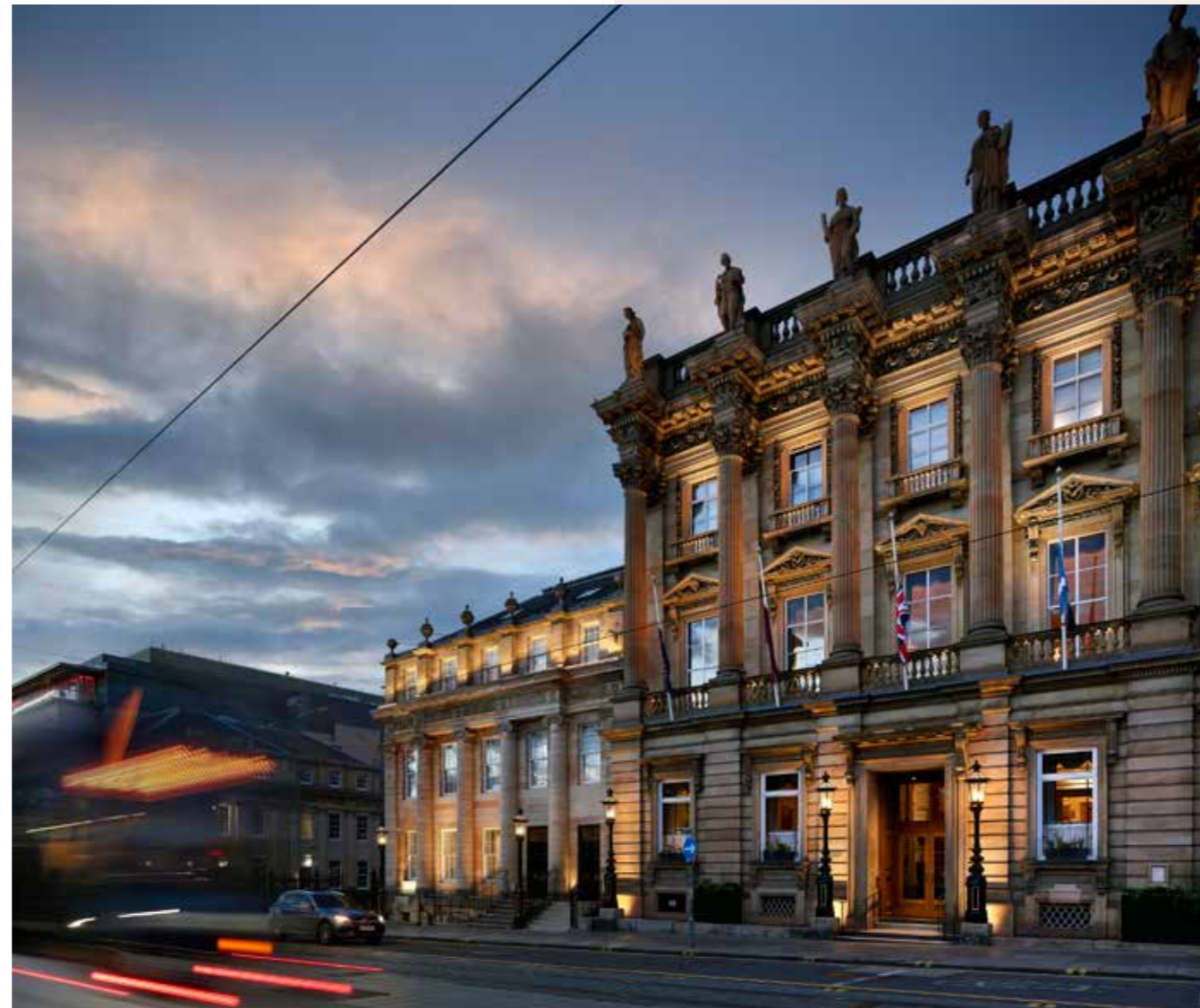
No. 39 St Andrew Square entrance.
